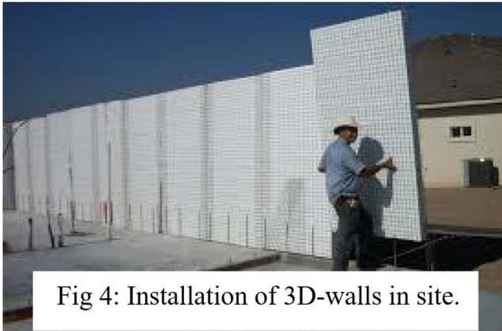
Figure 4: Installation of 3D-walls in site.
