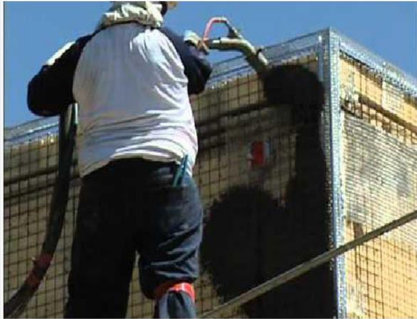
Figure 2: Coating of 3D-panel with shotcrete.
