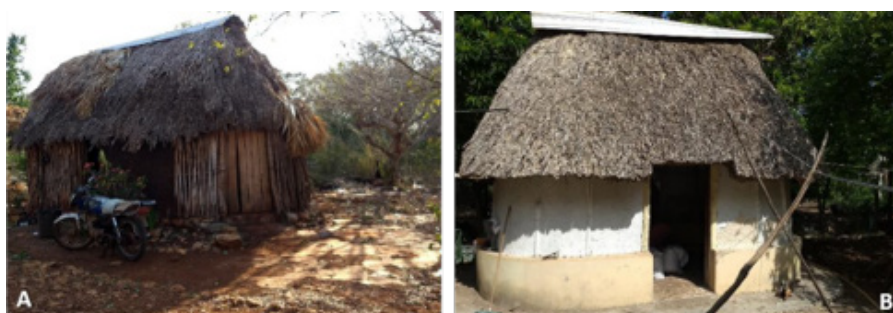
Figure 1: Mayan houses: A) Bajareque house with an apsidal floor plan with attached structures distributed in the center of the site, B) Masonry house with an apsidal plan.
