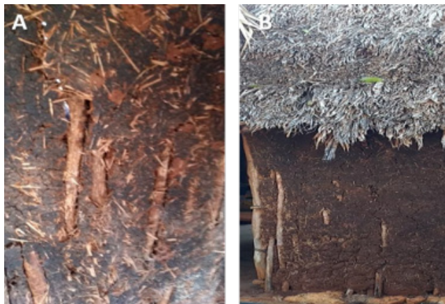
Figure 7: The application of the adobe mixture to the wall.
