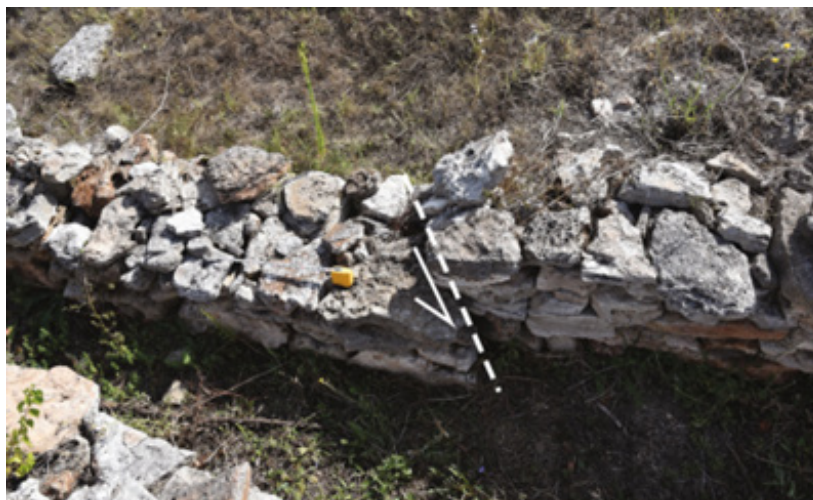
Figure 4: The seismic deformation on wall of a house built at the boundary between the Stone Age and the Copper Age - Island in Lake Durankulak (4450–4100 B.C.). This north–south wall has been fractured by strong seismic motion acting nearly parallel to the old wall [11]. Effects have been created by a strong earthquake of 4050 BC event.
