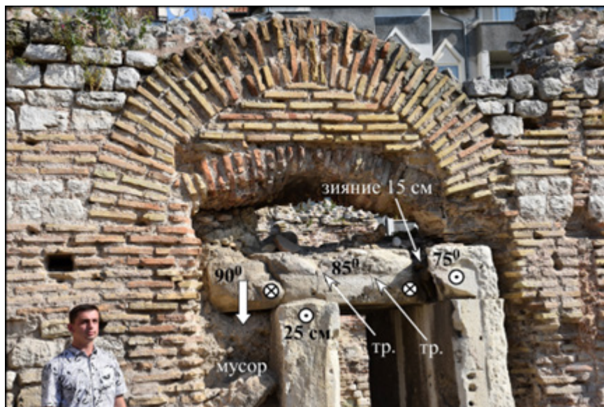
Figure 6: Entrance of the Frigidarium (Roma termi) affected by the strong seismic event. The numbers show azimuths of the cracks (tp.1 and tp.2). The shift of the horizontal stone bar is to the left. The vertical subsidence indicated by white arrow. This data gives the possibility to assess the direction of the seismic force as well as the power of it. Seismic event's source identified same as for the 6th c.AD [9].
