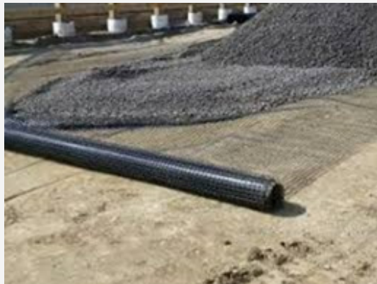
Figure 16: Permanent road by bituminous layer.
