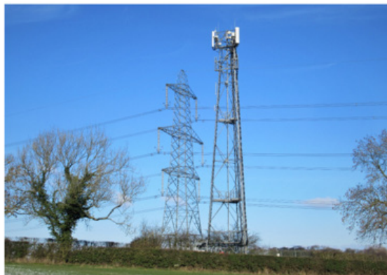
Figure 5: High voltage powerlines with a mast for microwave signals. A formidable combination. Easingwold; North Yorkshire; England. Photo by author.
