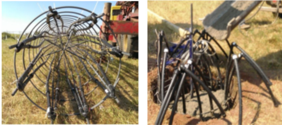
Figure 2: HDPE pipes attached to pile reinforcement [34].
