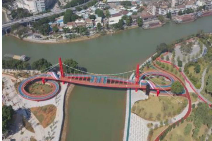
Figure 1: Xiasha pedestrian landscape footbridge.
