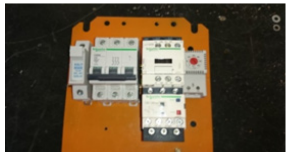
Figure 10: Assembling all components on Din Rail.
