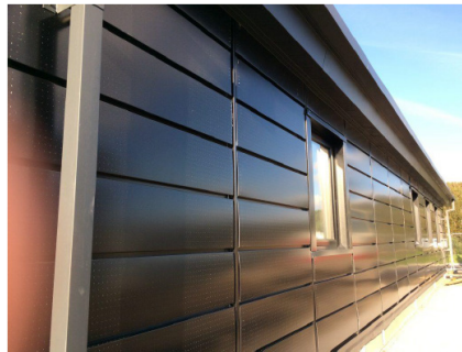
Figure 27: A Photovoltaic Thermal system on the south facing wall. The Source: Clarke, J. 2019
