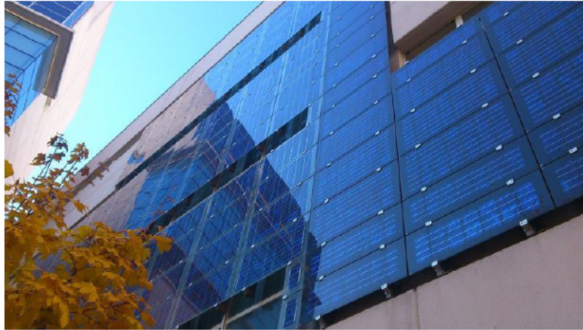
Figure 9: Using the Photovoltaic Panels on the façades to meet the building's energy needs. The Source: Zero Energy Project.
