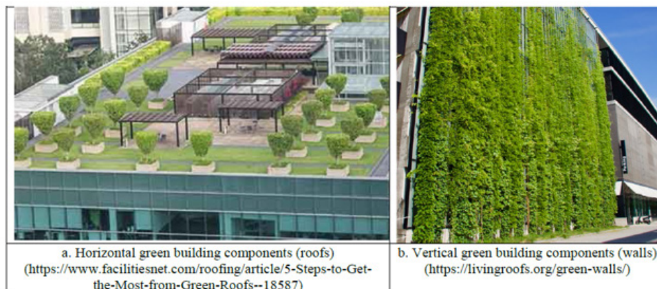
Figure 1: Greening systems: (a) Horizontal building components (roofs) & (b) Vertical building components (walls).
