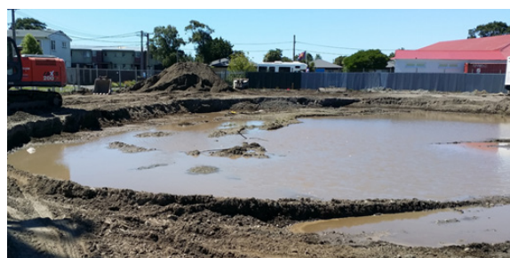
Figure 1: Shallow groundwater in an excavation for a retention basin in Christchurch.
