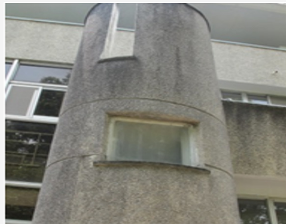
Figure 10: Washed finish after pouring concrete.
