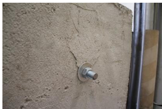
Figure 4f: Distinct spalling and detachment occurred at the bearing point – this was most clearly visible in the samples made of lightweight aggregate concrete.
