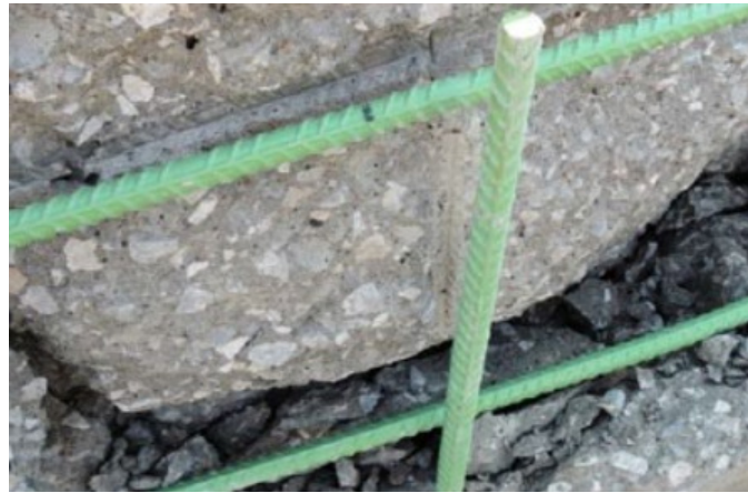
Figure 7: Lack of bond between epoxy-coated bars and concrete under impact loading.
