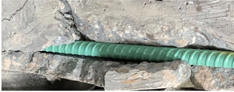
Figure 6: Lack of bond between epoxy-coated bars and concrete under static loading.
