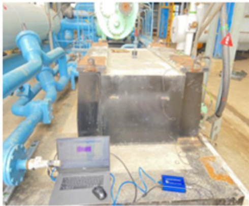
(a) Top middle signal acquisition of foundation
