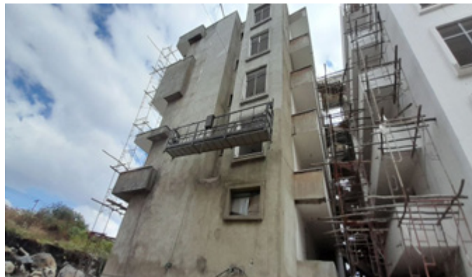
Figure 4: Suspended scaffolding system in Addis Ababa.
