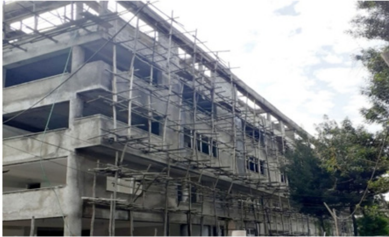
Figure 2: Wood scaffolding in public building projects in Addis Ababa.
