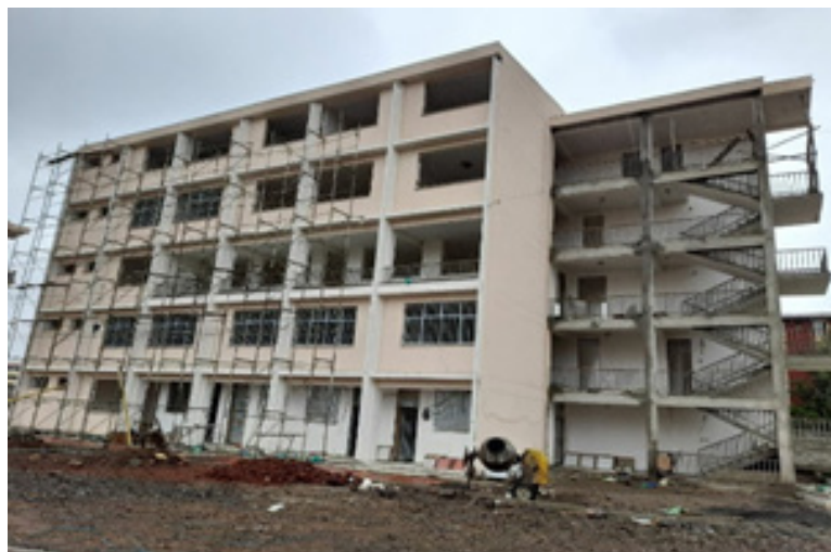
Figure 3: Metal scaffolding in public building projects in Addis Ababa.
