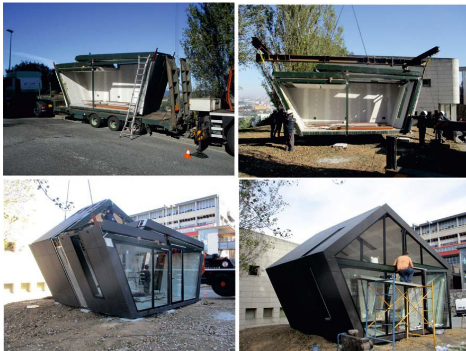
Figure 7: Module installation phases.
