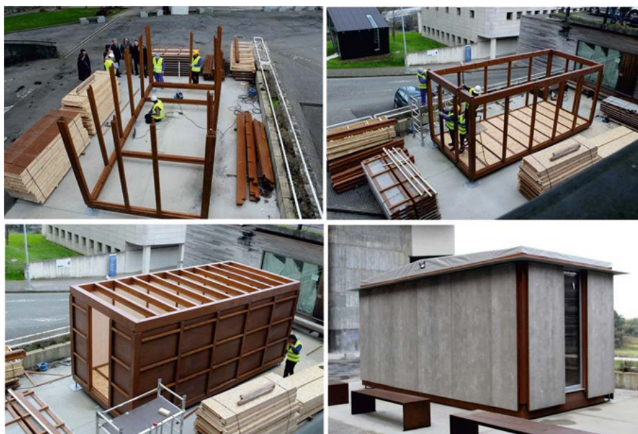
Figure 11: Module assembly phases.
