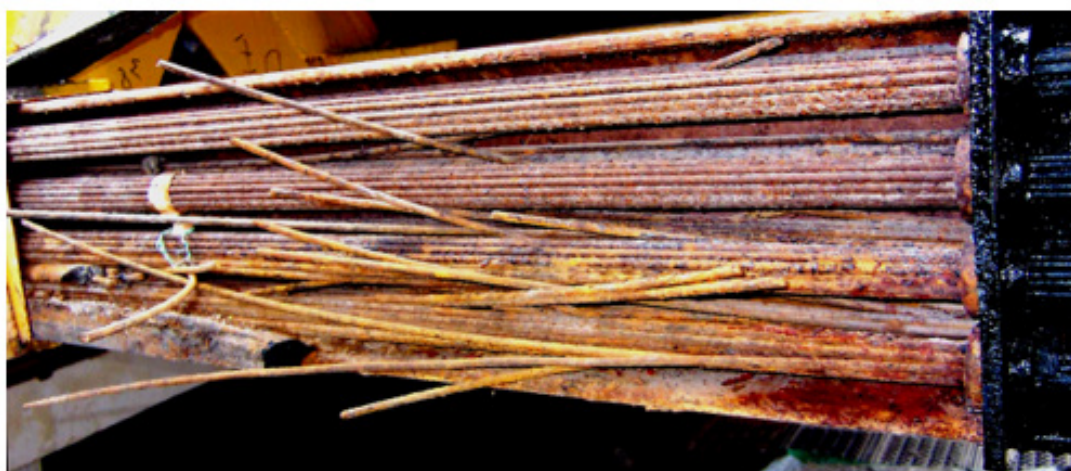
Figure 3: Example of damage to girder prestressing tendons [own study].
