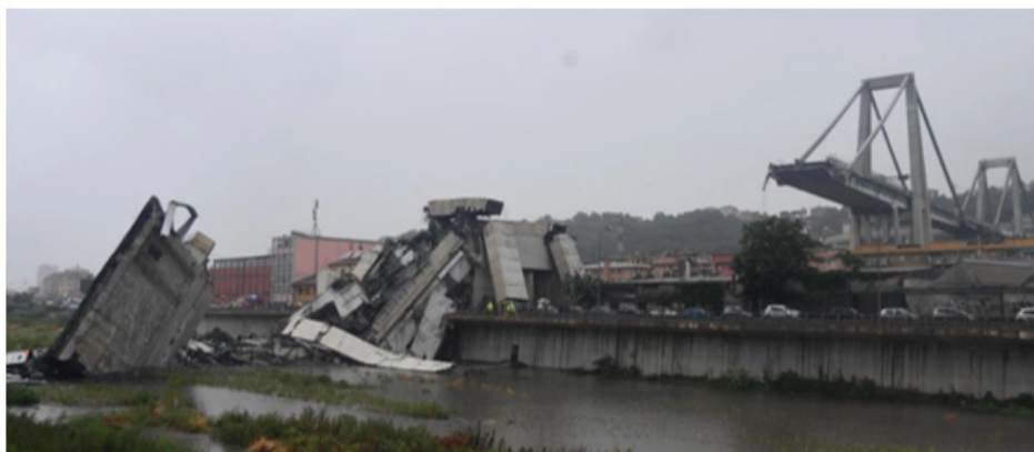
Figure 4: Collapsed bridge in Genoa (2018) with visible ruptures of steel prestressing tendons [own study].
