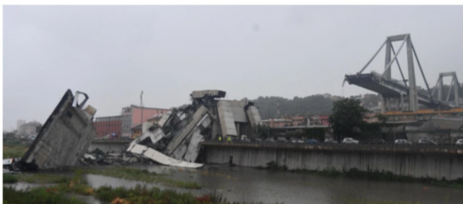
Figure 4: Collapsed bridge in Genoa (2018) with visible ruptures of steel prestressing tendons [own study].
