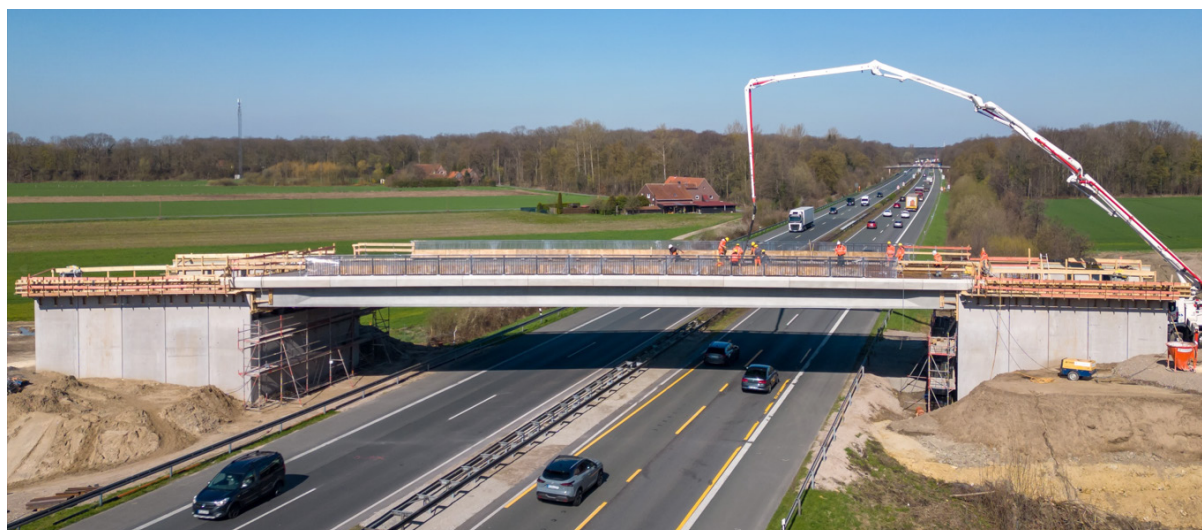
Figure 8: Concreting of the in-situ concrete layer under running traffic, Amelsbürener Straße structure.
