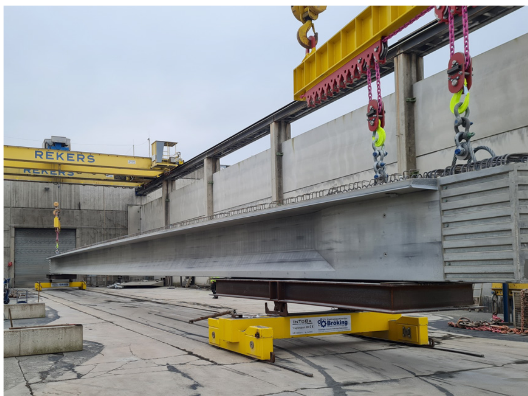
Figure 5: Removal of the precast girders after production in the precast plant.
