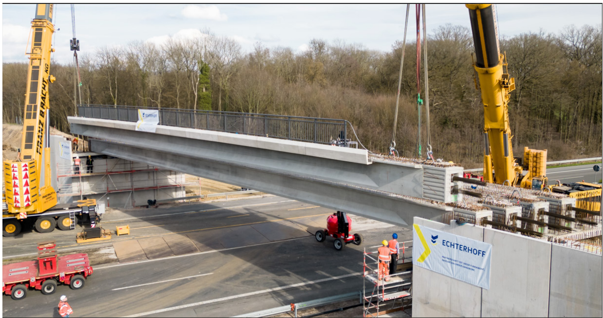
Figure 7: Lifting in of an edge beam with pre-assembled carbon cap and railing, Amelsbürener Straße building.
