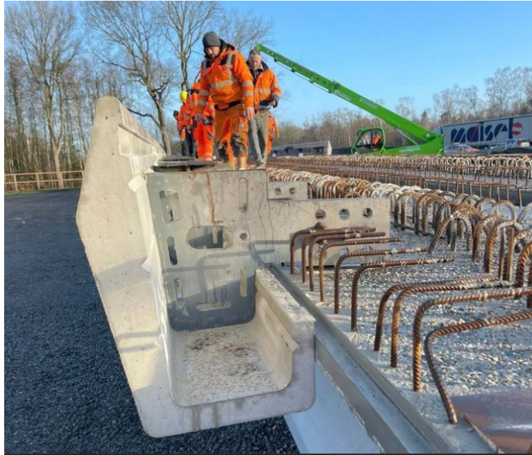
Figure 6: Panel of carbon concrete (system of the Echterhoff Group), Amelsbürener Straße building.
