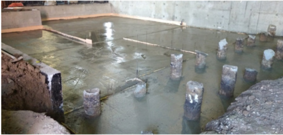
Figure 2: Fragment of ERT bored injection pile outlets.
