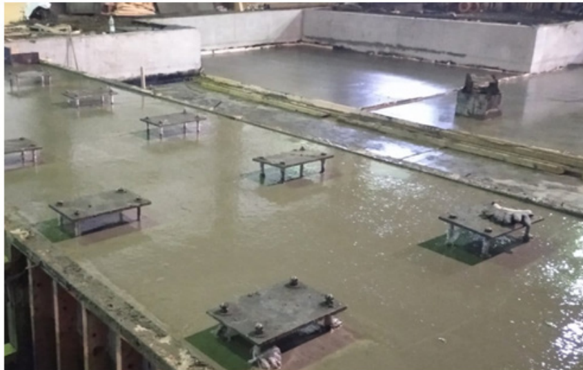
Figure 3: A fragment of a ready-made monolithic reinforced concrete structure for the installation of super-foundation structures and equipment.
