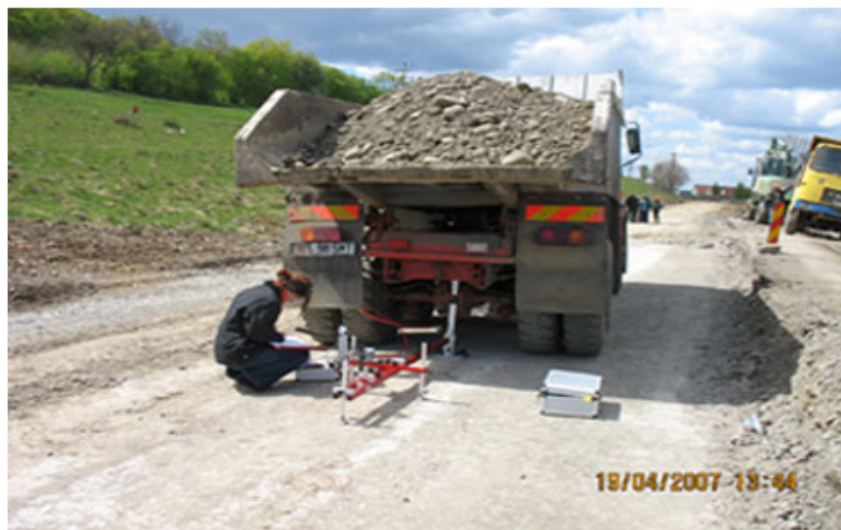
Figure 4: Loading the Lucas plate using a heavy truck (source: ILFA CON SRL).
