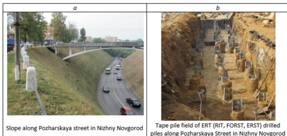
Figure 2: Tape pile field of ERT (RIT, FORST, ERST) drilled piles along Pozharskaya Street in Nizhny Novgorod.
