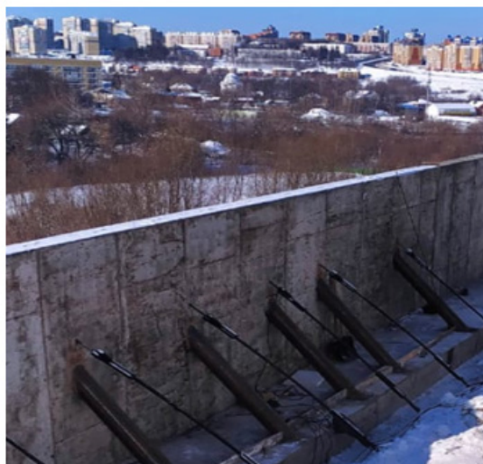
Figure 3: Recessed retaining reinforced concrete structures using ERT bored piles (RIT, FORST, ERST), ERT ground anchors and monolithic reinforced concrete corner retaining walls in Cheboksary.
