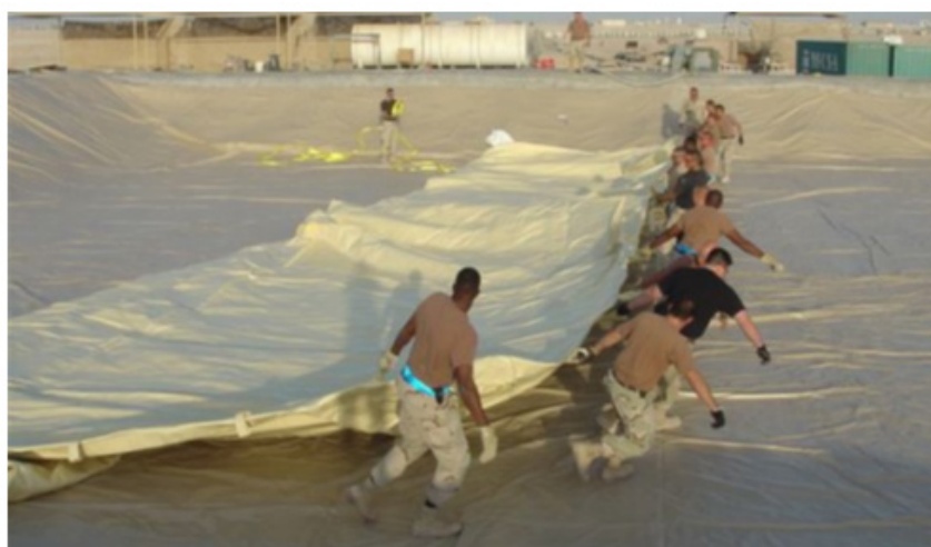
Figure 8: Preparation of flexible tanks for use [26].
