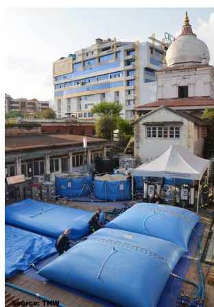
Figure 11: WTC 5000 UF water treatment and storage system in Kathmandu. Source: Federal Agency for Technical Relief (THW, Germany)
