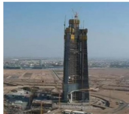
Figure 1: Jeddah tower, a one-kilometre-tall concrete building (under construction).
