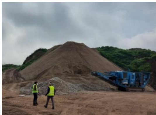
Figure 2: CDW plant with stockpile of recycled material with possible application in concrete.
