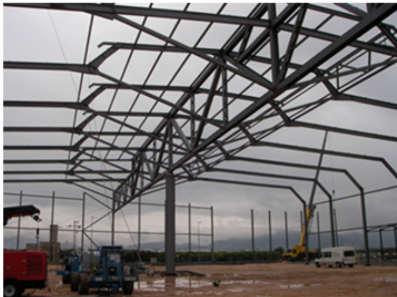
Figure 5: General view of warehouse I structure during erection.
