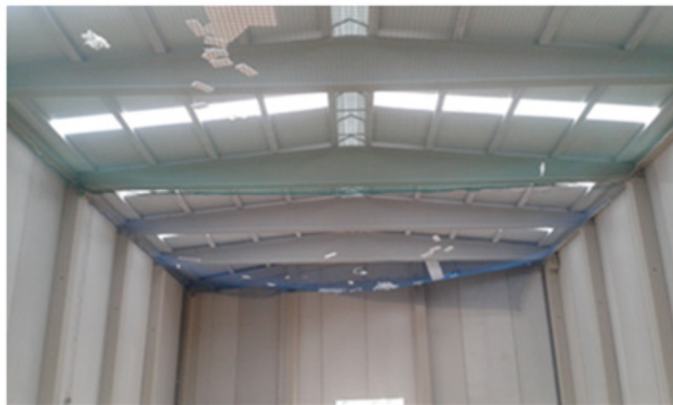
Figure 8: Interior view of the packaging warehouse during construction.
