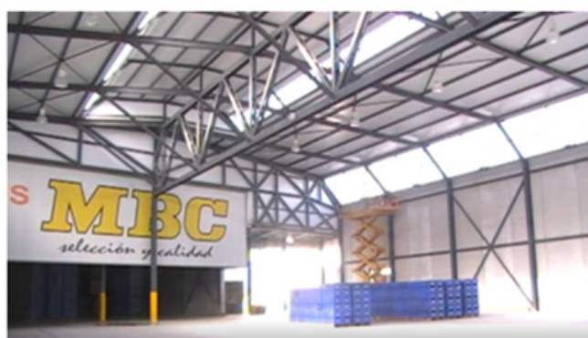
Figure 9: Interior view of warehouse III after it was just built.
