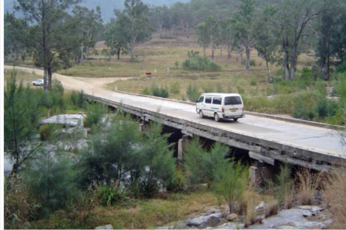
Figure 1: Mann River Bridge, Wyaliba Bridge before fire (Glencross-Gant, 30 April 2007).
