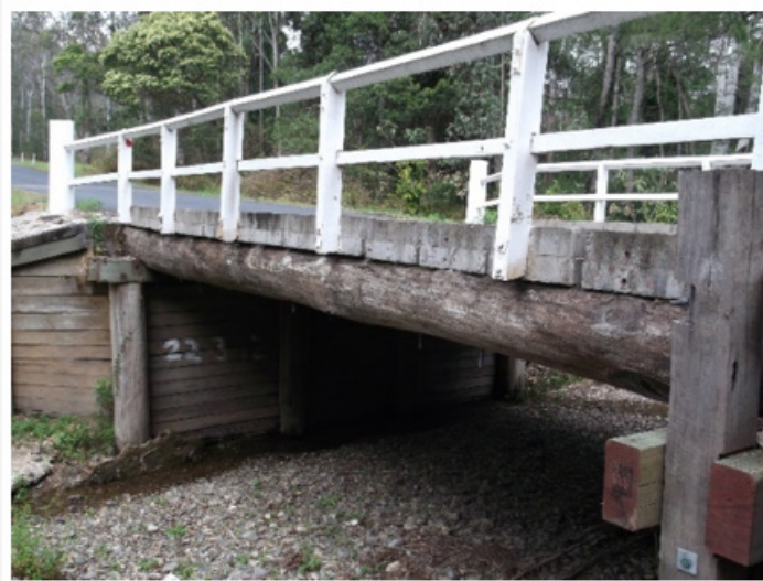
Figure 5: Single span timber Beam Bridge over Hortons Creek (Glencross-Grant, 8 December 2013).
