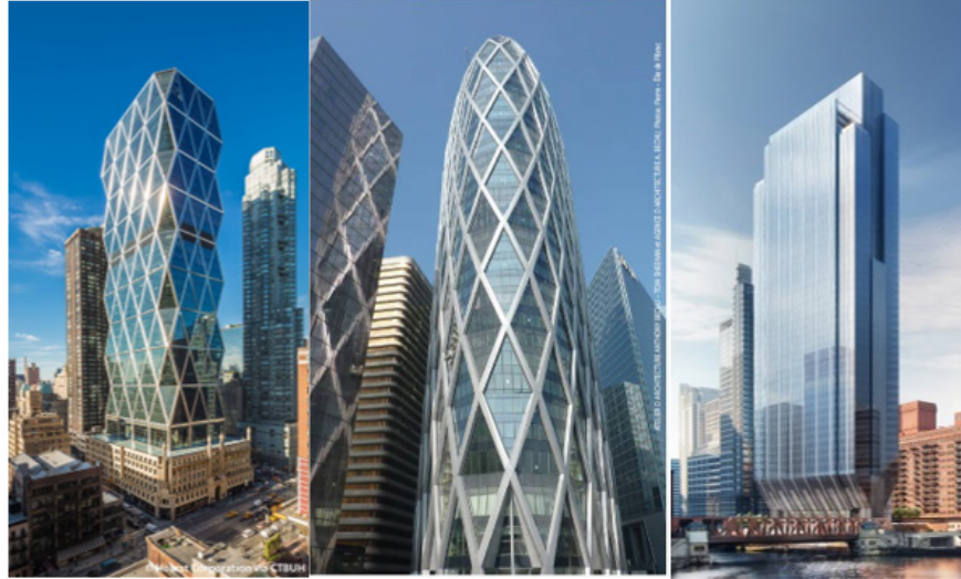
Figure 3: Left: Hearst Tower in NYC (USA) @Hearst Corporation; Center: Tour D2 in Paris (France) @ Atelier Architecture Anthony Bechu; Right: 150 N Riverside, Chicago (USA) @ Goettsch Partners.
