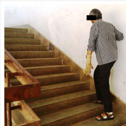
Figure 2: An individual with stroke and left hemiplegia finds unavailability of rails on right side while climbing stairs as a barrier
