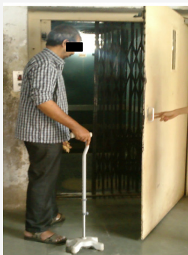
Figure 4: Cramped and heavy doors of the lifts perceived as a barrier
