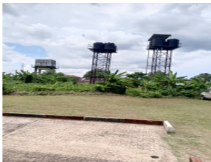
Figure 3: Abandoned borehole in Ibeno (Government-funded project).
