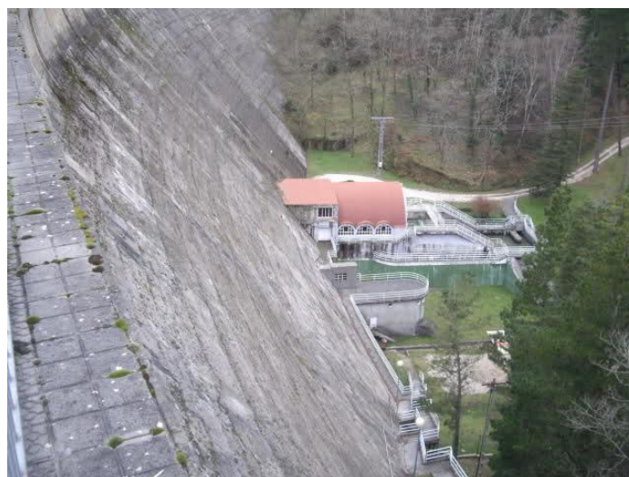
Figure 5: Photograph of the dam-toe Ordunte HPP
